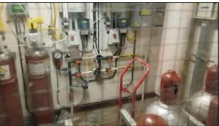
The vacuum regulating injection system used chlorine gas from compressed cylinders with an automatic switchover system. The compressed gas is injected into the water system via the Series V10 chlorinator and injector.
