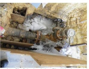
due to a lack resistance to lateral movement due incomplete fill of the insulation fill within the metal enclosure. Lateral displacement of the piping could lead to separation of the couplings on the AC piping. It has also been noted that the valve at the trust block represents vulnerability due to freeze or vandalism.
