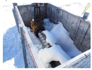
The watermain extends beyond the thrust block within a metal enclosure. Access into the metal enclosure between the trust block and the northern most row house block was very limited due to snow cover over the enclosure. The metal enclosure within 9 meters of the thrust block has been repaired with a wooden cover. City staff opened this wooden cover, which provided the opportunity to determine that the piping near the trust block is 200 mm iron pipe.
