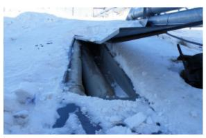
It was reported that most of the piping situated between the row housing units is AC. This could not be confirmed as much of the enclosure is covered with gravel and snow. The condition of the metal enclosure, at those locations where the enclosure is visible, supports this report.
