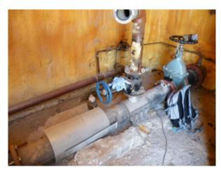
the thrust block. A pair of repair clamps has been installed on the HDPE piping within 4 metres of the trust block. The plywood enclosure surrounding the valve is in an advanced state of deterioration leaving the valve poorly enclosed and at risk of freeze and vandalism. This valve is currently not essential for operational reasons, as this function can be provided by the valve situated upstream in the metal building. Photographs below depict the arrangement in the vicinity of the thrust block.
