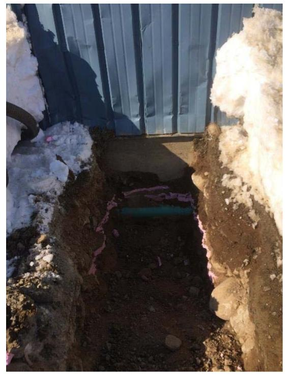
Photo A3: Test Pit adjacent to Existing Building, i.e. TP-2 (Note Green PVC Pipe and Insulation)
